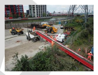
live Signalling, Fibre and LV cables separating our compound and the only access point to the site of work. Conveyors were then used to transfer 1600t of old track ballast and return new into the site, all the S&C and plain had to be built loose and the entire layout tamped by hand as we had no way to access tampers into the site.
